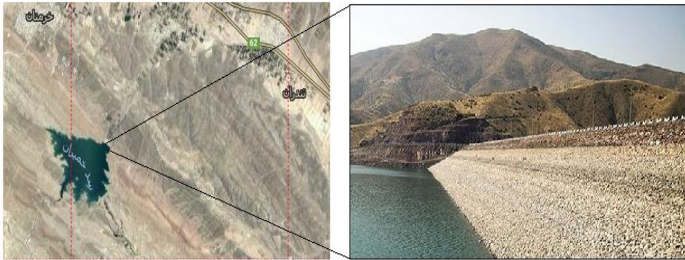
Figure 7) the location of Khamiran dam on Khamiran river
