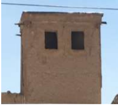
Figure 3) a) Two-way wind catcher in Shariat Panahi house
